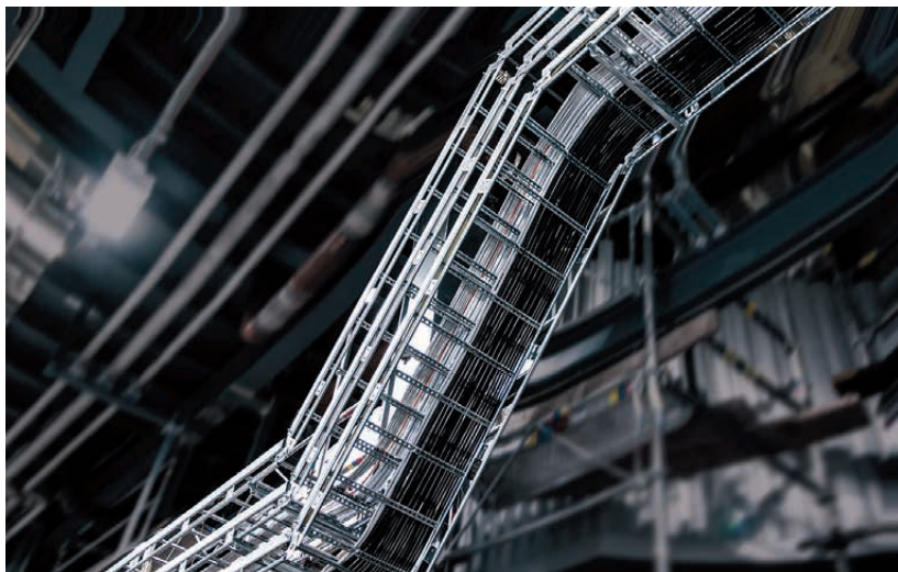
Figure 7. Cable ladder manufactured using a special tube profile. Courtesy of Meka Pro Oy.
